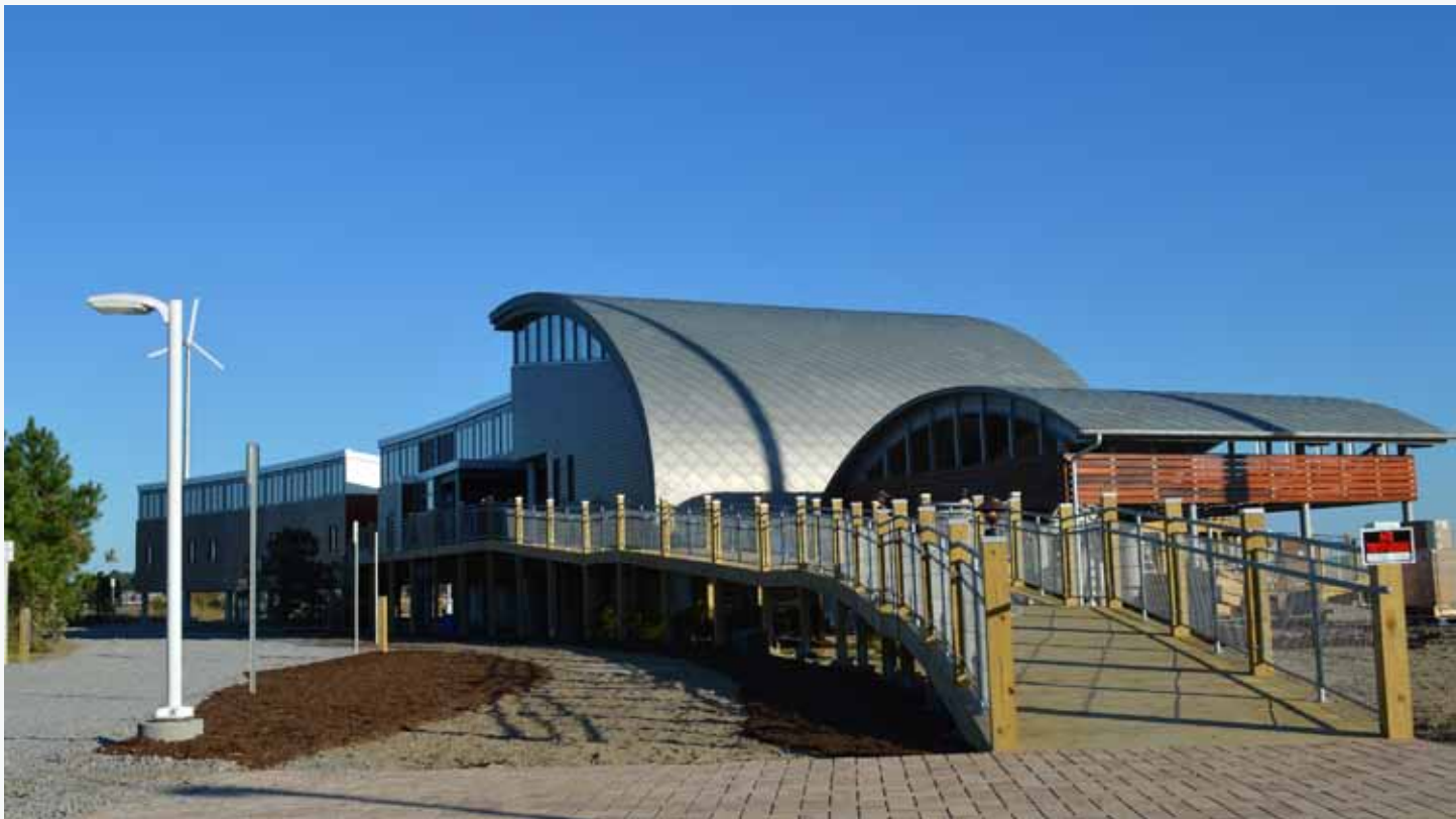
The Chesapeake Bay Foundation hopes that the building will become the first LEED Platinum-certified project in Virginia.
